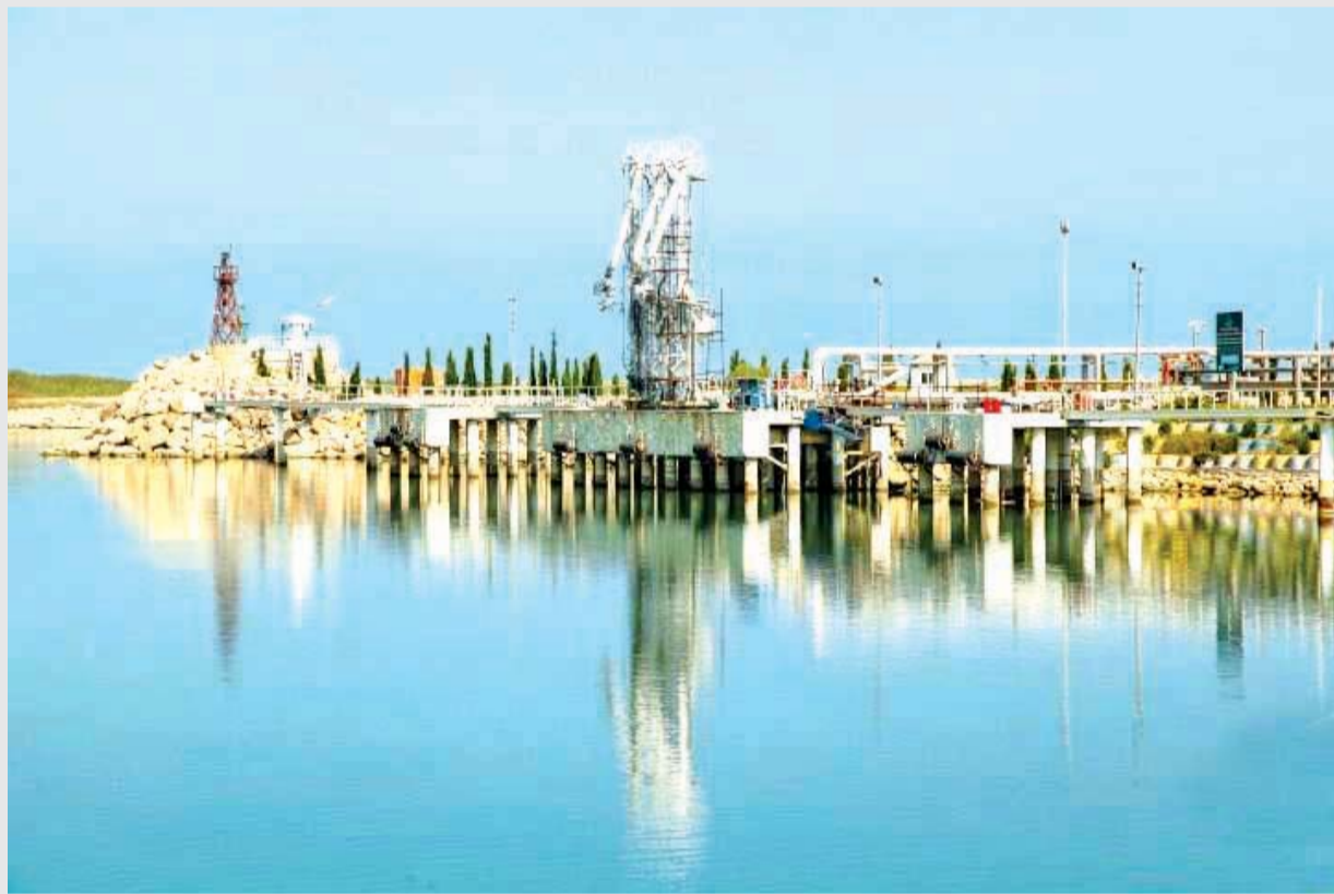
Iran's modern North Oil Terminal located in the northern city of Neka has been established aiming to receive, store, process and transport crude oils of Caspian Sea marginal states under SWAP (exchange) plan. The project is planned to be completed in three phases, it will have the capacity of receiving and transferring 50000, 120000 and 370000 barrels per day (bpd) of oil, in the first, second and third phases respectively.
