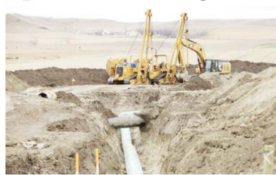
Construction equipment sits near a Dakota Access Pipeline construction site off County Road 135 near the town of Cannon Ball, North Dakota, U.S. on October 30, 2016.
