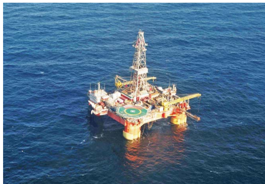
Amir Kabir semi-submersible drilling rig in the Caspian Sea, north of Iran
