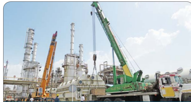
Installing Filters in Waxing Unit
