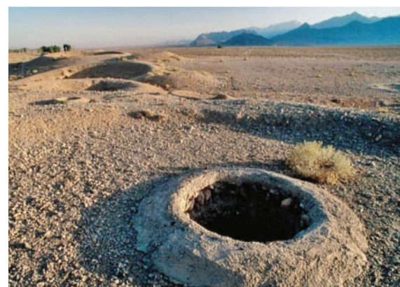
Anthill-like shafts were bored into the earth to reach underground water sources
