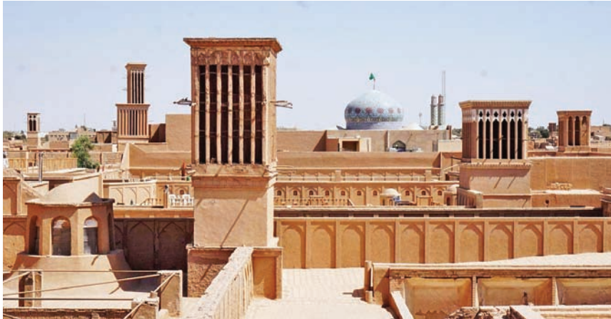
For centuries, badgirs (wind catchers) have helped Yazd residents stay cool despite desert temperatures that can reach 40C in summertime (Credit: Shervin Abdolhamidi)
