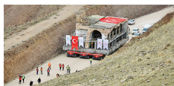
The Er-Rizk Mosque is being moved from Hasankeyf, which is going to be flooded because of construction of the Ilisu dam, to the new Hasankeyf Culture Park
