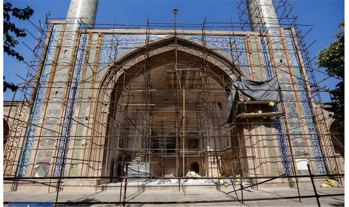
A portico of the Jameh Mosque of Qazvin is seen behind scaffolding in an undated photo.
