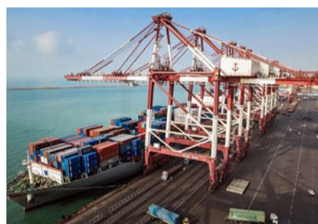
20) and said about 900 meters of docks at the phase three of container part will be completed
