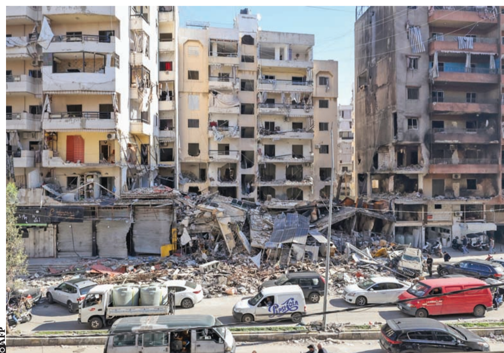
Cars drive past buildings that were damaged or destroyed in Israeli strikes in Beirut's southern suburbs Hay el-Sellom neighborhood on December 2, 2024.
