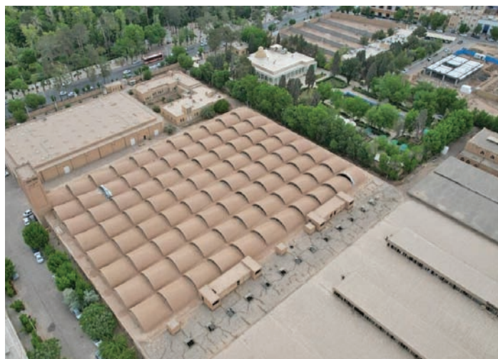
An aerial view of the Janoub textile factory located on Ayatollah Kashani Street in Yazd, central Iran.
