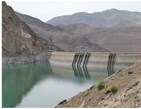
Fars, Tangouyeh Dam in Sirjan, Kerman Province, and Saveh Dam in Markazi Province.
