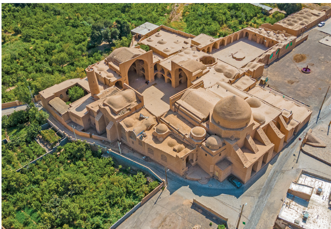
An aerial view of the Jameh mosque of Ardestan located in the north of Isfahan province, central Iran.
