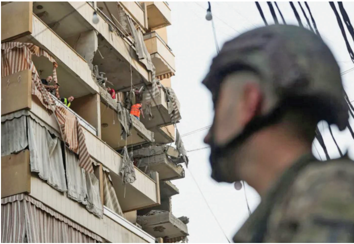
A building damaged by Israeli strikes in southern Beirut on November 23, 2025.
