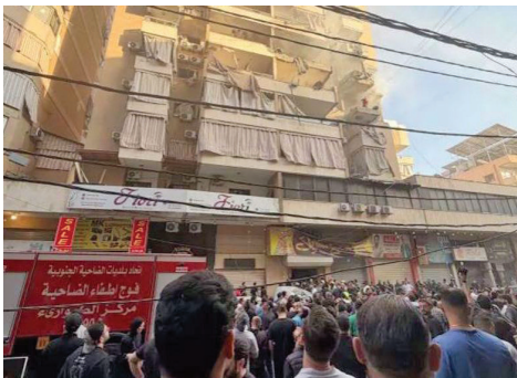
A crowd gathers below a damaged residential building following an Israeli military strike in southern Beirut's Haret Hreik neighborhood on November 23, 2025.
