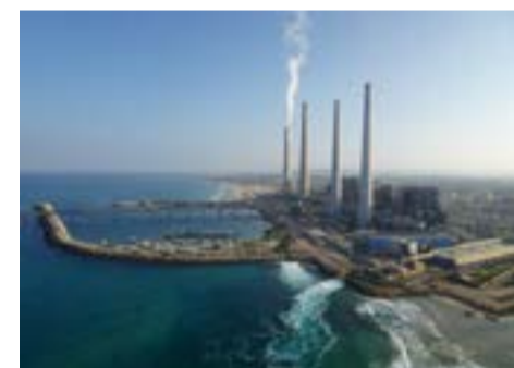
Orot Rabin is Israel's largest power station, representing about 20% of the regime's total generation capacity
