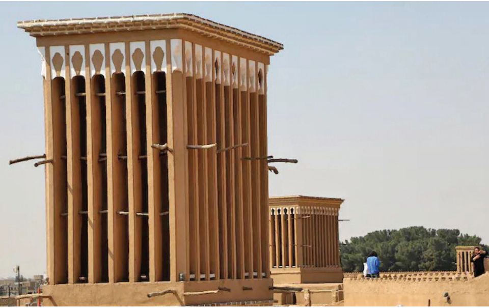
Windcatchers or wind towers are traditional architectural elements have been used to create cross ventilation and passive cooling in buildings in Iran for centuries.
